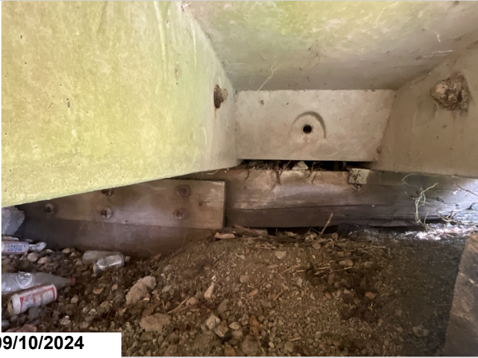
Abutment 2 Cap, Right End, Last 6': Decayed with heavy section loss and crushing up to 2" onto pile 6. Approximately 20% remaining.
