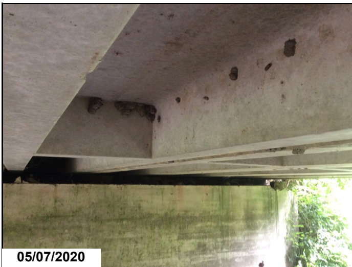
Typical missing bolt at center span.
