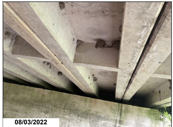
Both Connection Bolts, Center Span, Between Units 5 & 6: Missing. Connection Bolt, 3/4 Span, Between Units 6 & 7: Missing. Connection Bolt, Center Span, Between Units 6 & 7: Backed out.
